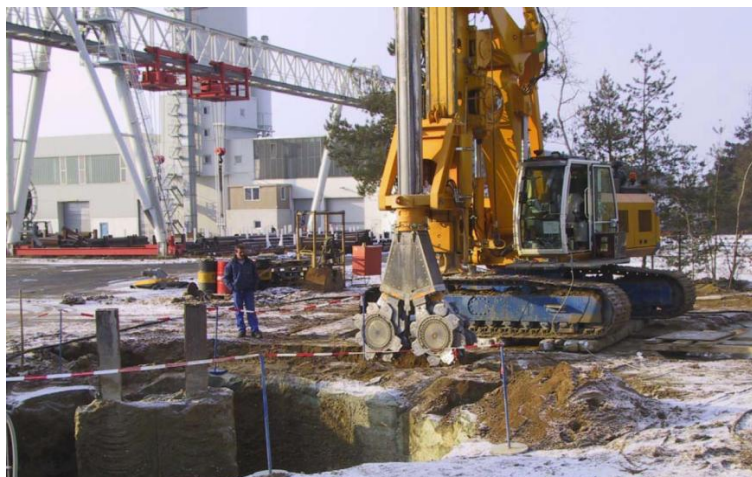
Figura 21 - Attrezzatura CSM (Cutter Soil Mixing)
